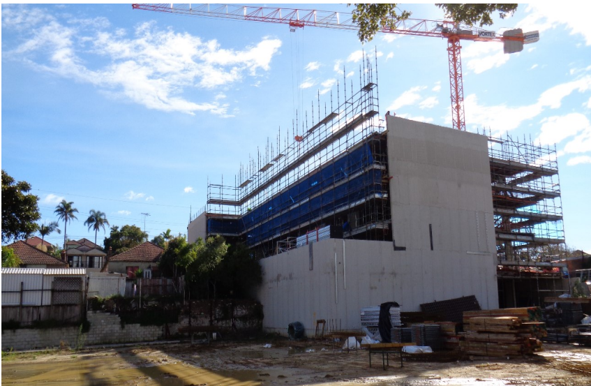
Figure 4 - Development under construction to the north east and semi's to the rear
